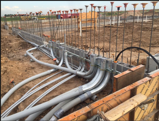
Slab rough-in at Ninnescah REC building in Pratt.
