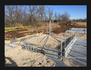
Foreman Brent Combs and his crew will complete the slab rough next week to prepare for the concrete slab. The project should be completed in September of 2017.
