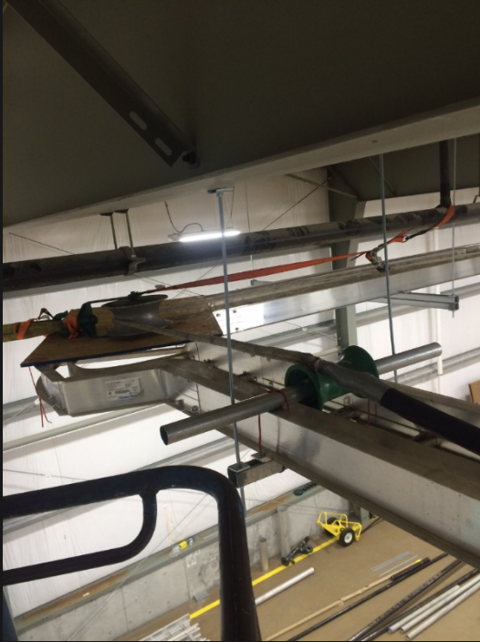
Pulling wire at the KanPak plant in Arkansas City. Foreman, Kyle Kennedy
