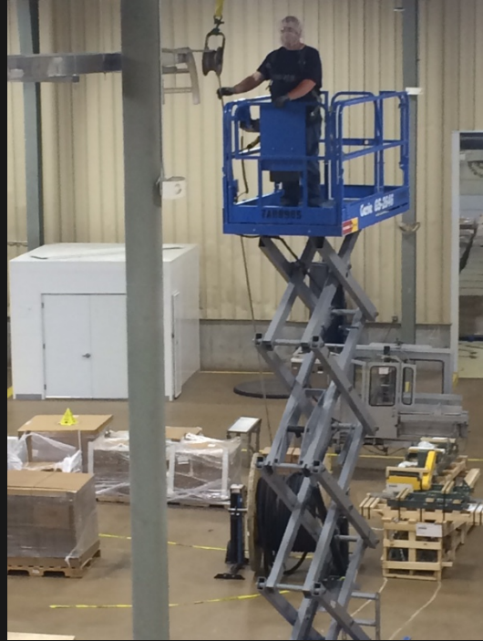
Pulling wire at the KanPak plant in Arkansas City. Foreman, Kyle Kennedy
