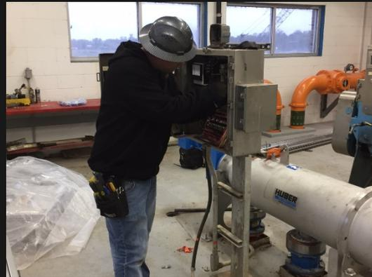
Jason DeBerry and Eric Phelps have been working at the City of Wichita Sewer Treatment Plant #2. Decker Electric worked on the Clarifier Drive Replacement and the demolition and replacement of the screener control panel and air compressor hook-up.
