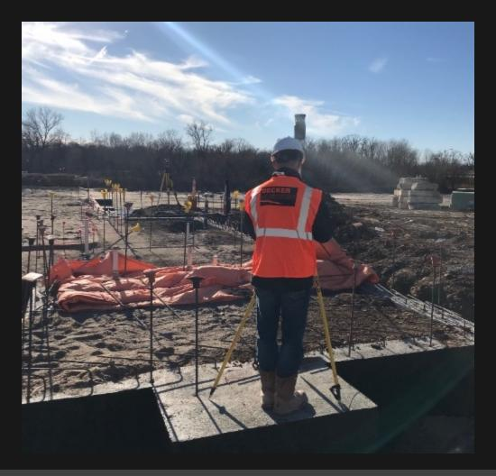
Using our Trimble Robotic Total Station (RTS) as a live link between design documents and the construction site has been a great success to being more efficient and accurate with layout and accelerating construction activities.
